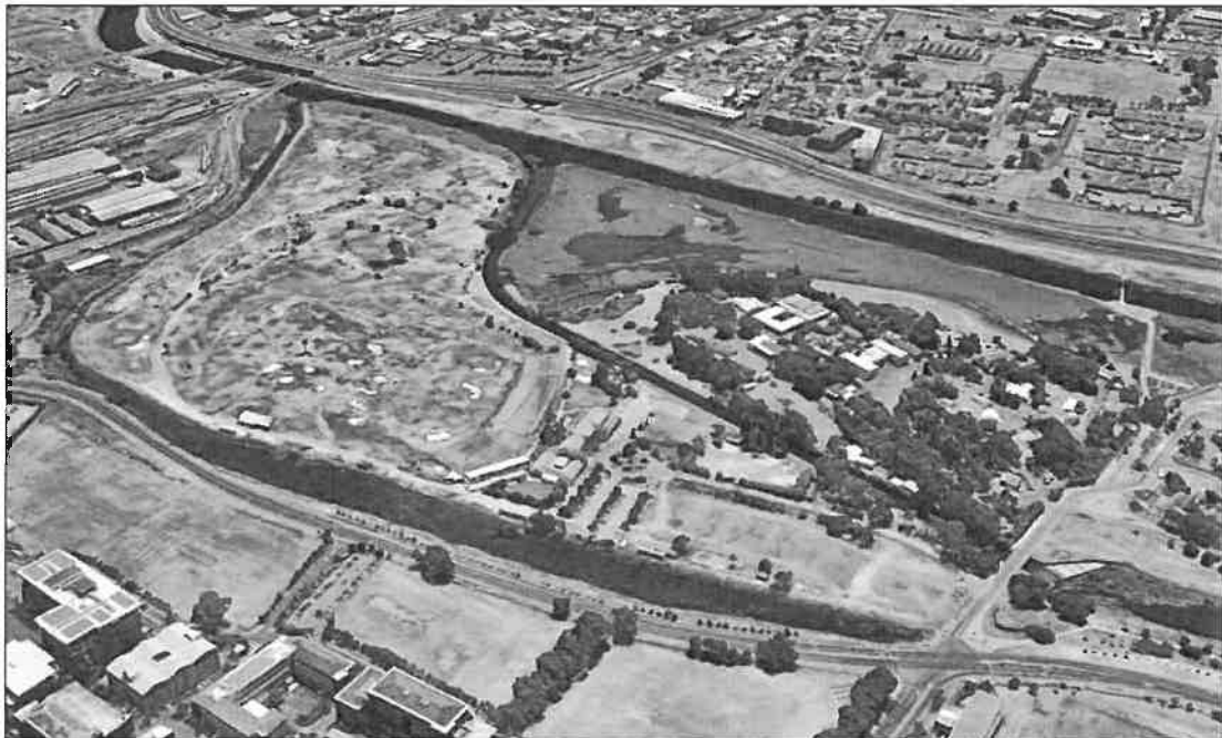
Figure 2: Aerial view of the site and environs
