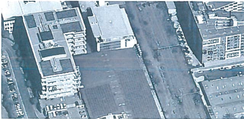
Black River Business Park buildings heights approximately 23m
