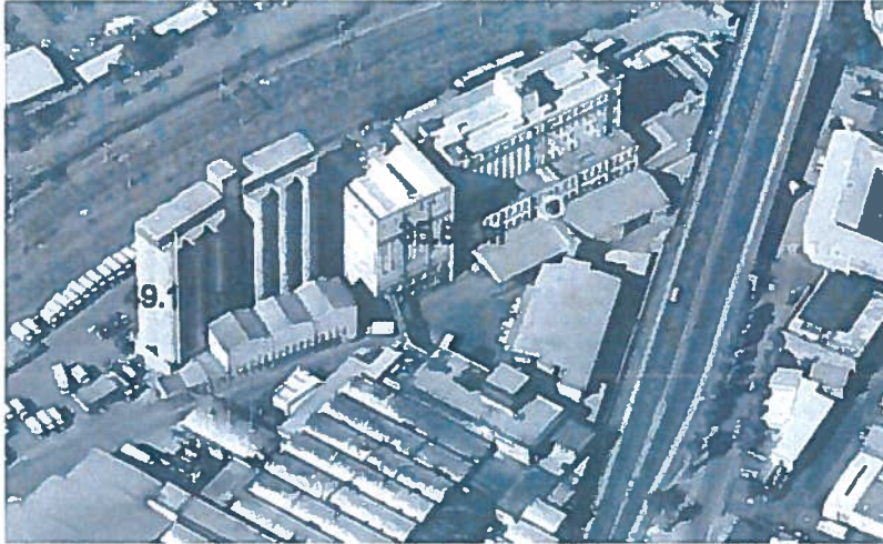
Premier foods building heights in Salt River approximately 36m (bins about 49m)
